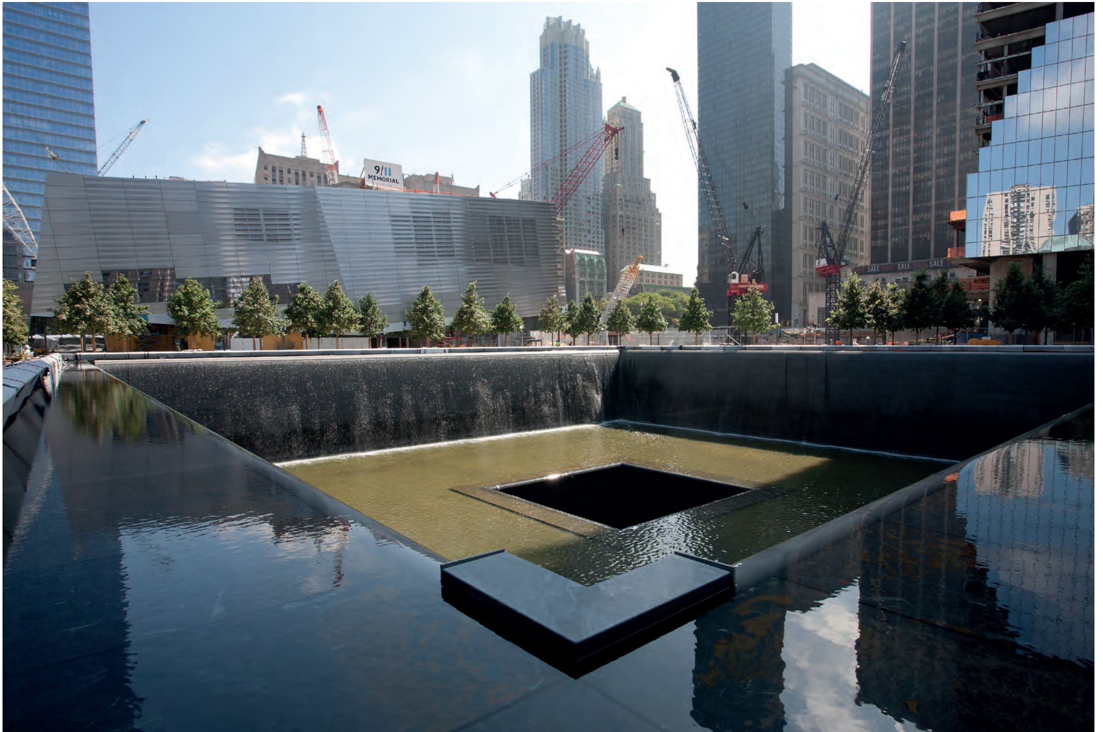
The 9/11 Memorial Fountain, Lower Manhattan (under construction) Photograph: Amy Dreher
