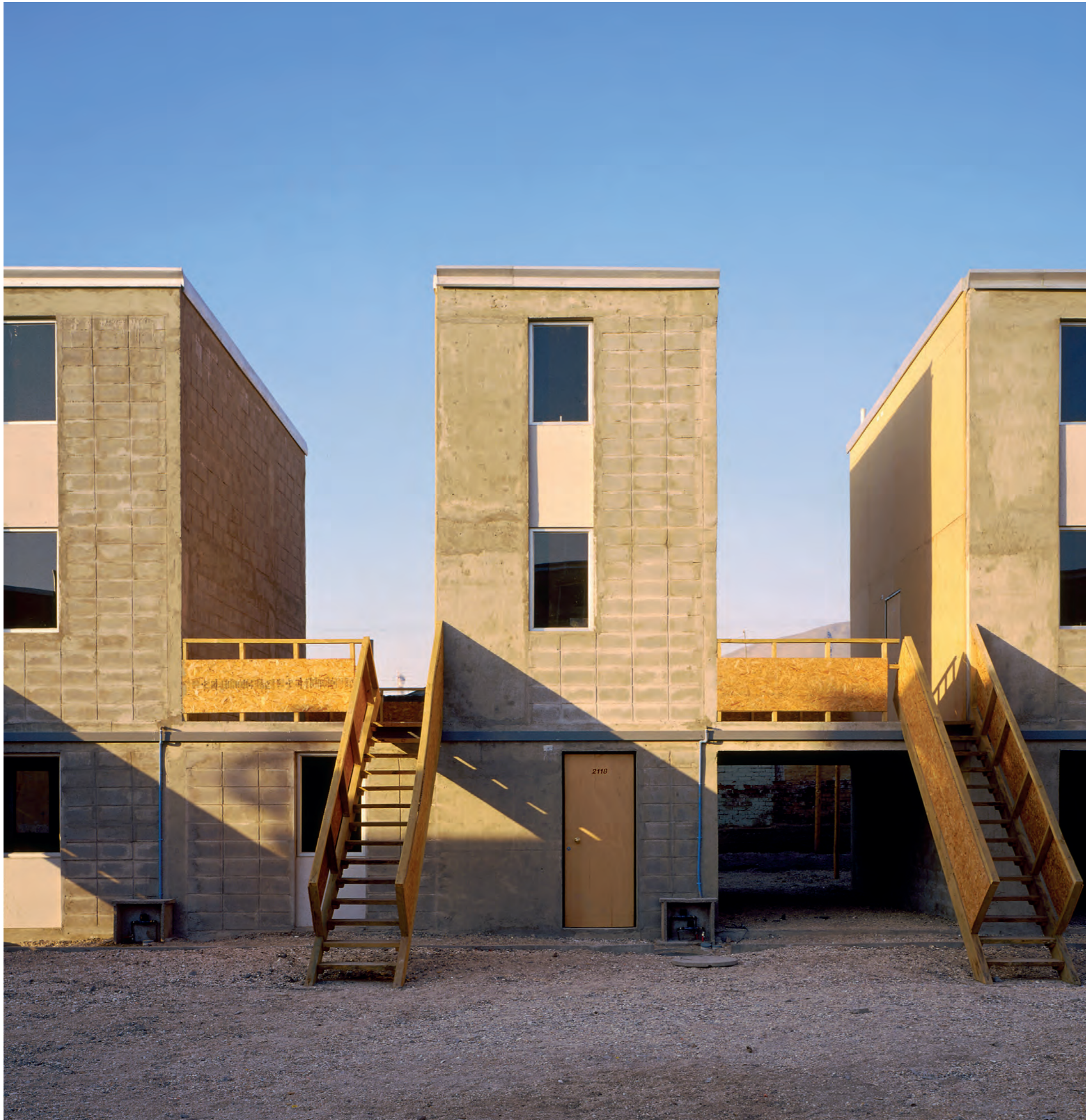
The Incremental Housing project in Iquique, Chile and Monterrey, Mexico produces half-finished houses that are completed by the residents and contain only the essentials of a built home – bathroom, kitchen, structure and roof – in order to stretch resources further to meet the rapidly growing demand for housing Architects: Alejandro Aravena, Tomás Cortese, Emilio de la Cerda, Andrés Iacobelli and Alfonso Montero, Elemental (Chile); engineers: José Gajardo, Juan Carlos de la Llera; urbanization specialist: Proingel and Abraham Guerra. Construction: Loga S.A. Client: Chile Barrio. Iquique, Chile, 2003-4. Concrete, brick concrete, wood panels Photograph: Elemental
